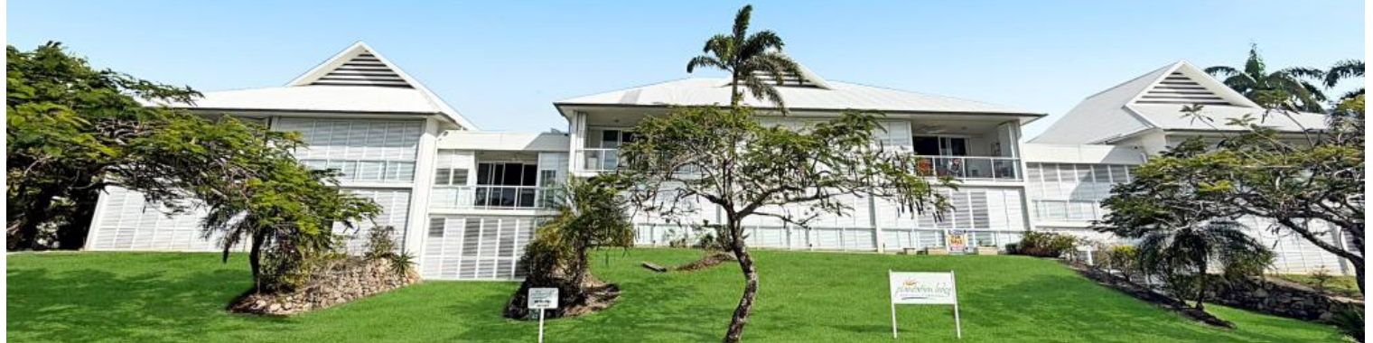
Unit 13, 20-24 Poinciana Boulevard, Cardwell
